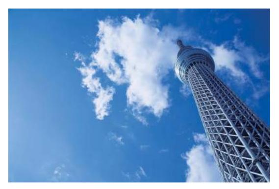
'Sky tree' the new land mark of Tokyo is 634m high and much higher than previous land mark 'Tokyo Tower' 'Sky tree', such a high tower is realized by applying the steel pipe structure
